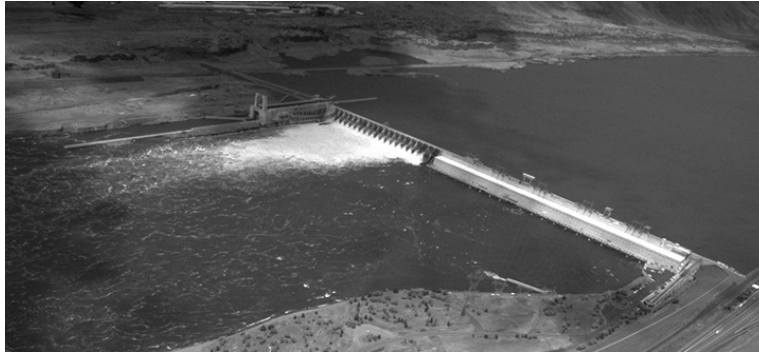
Figure 1.1. Aerial Photograph of John Day Dam. Flow is from right to left.
